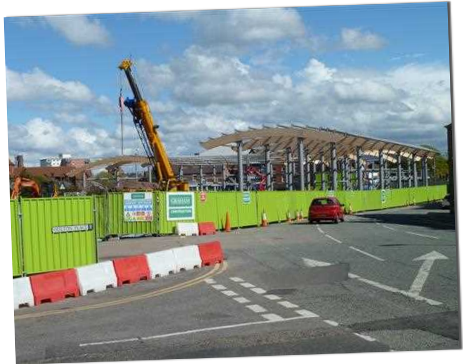
Chester's New Bus Station under construction. On the old cattle market.
